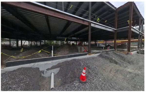
Underground Sanitary and Storm piping installation and inspections are underway. Backfilling operations continue as other MEP underground layout and install takes place. Steel erection was completed with the final beam topping off ceremony. Students and faculty signed the beam, and it was raised into place. This marks a major milestone in the construction of the new middle school.
